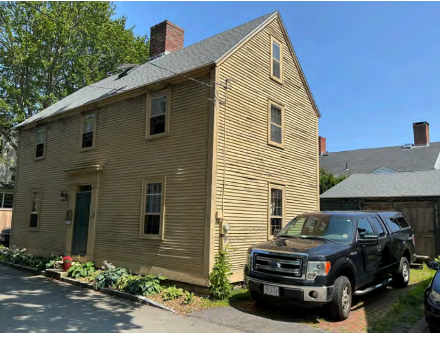
EXISTING CONDITION PHOTO
