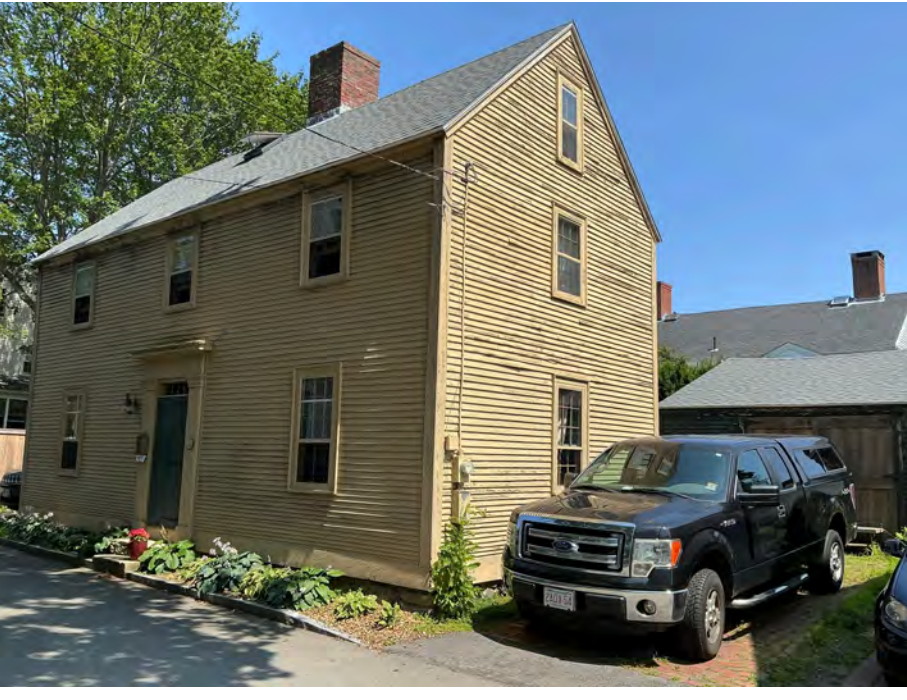
EXISTING CONDITION PHOTO
