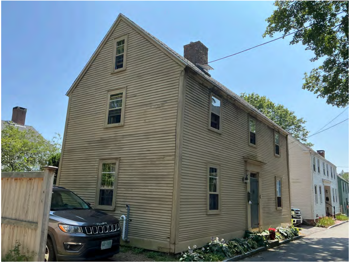
EXISTING EAST VIEW
